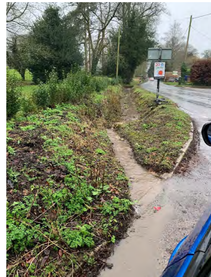
Figure 5: The ditch-like winterbourne headwaters of the Candover Brook taking road run-off during a heavy rainfall event.
