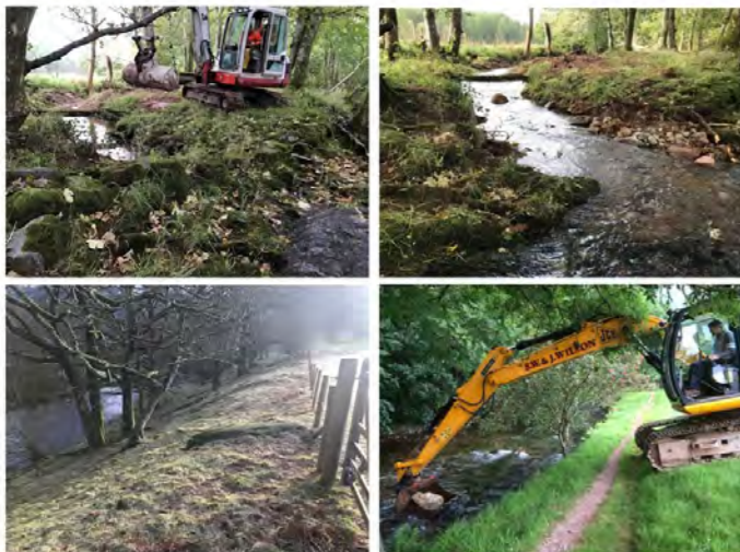
Figure 3: Restoration activities carried out by WCRT include re-connecting paleo-channels (top left and right before and after respectively), fencing the river bank to create buffer strips (bottom left) and replacing boulders in the river to increase habitat diversity (bottom right).
