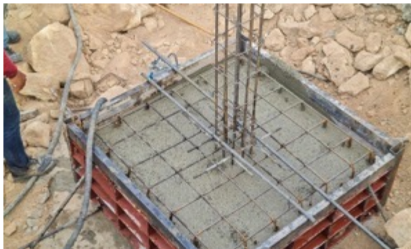
Concrete reinforced with steel bars (rebar)
