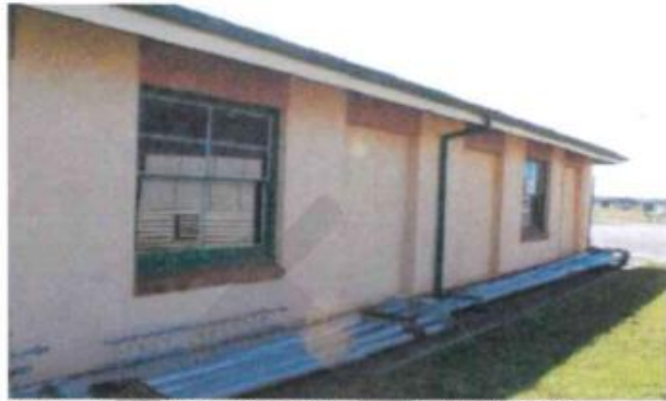
Figure 2: Eastern elevation of the Shell Kiosk (AHS 2021).
