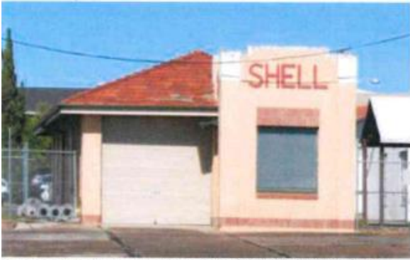
Figure 1: Northern elevation of the Shell Kiosk (AHS 2021).
