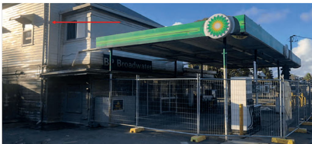
Figure 11: The approximate height of flood water (red arrow) against a still-closed Broadwater service station (top) and some of the many flood-deposited vehicles from over two weeks earlier. (Photo courtesy of Risk Frontiers 2022)
