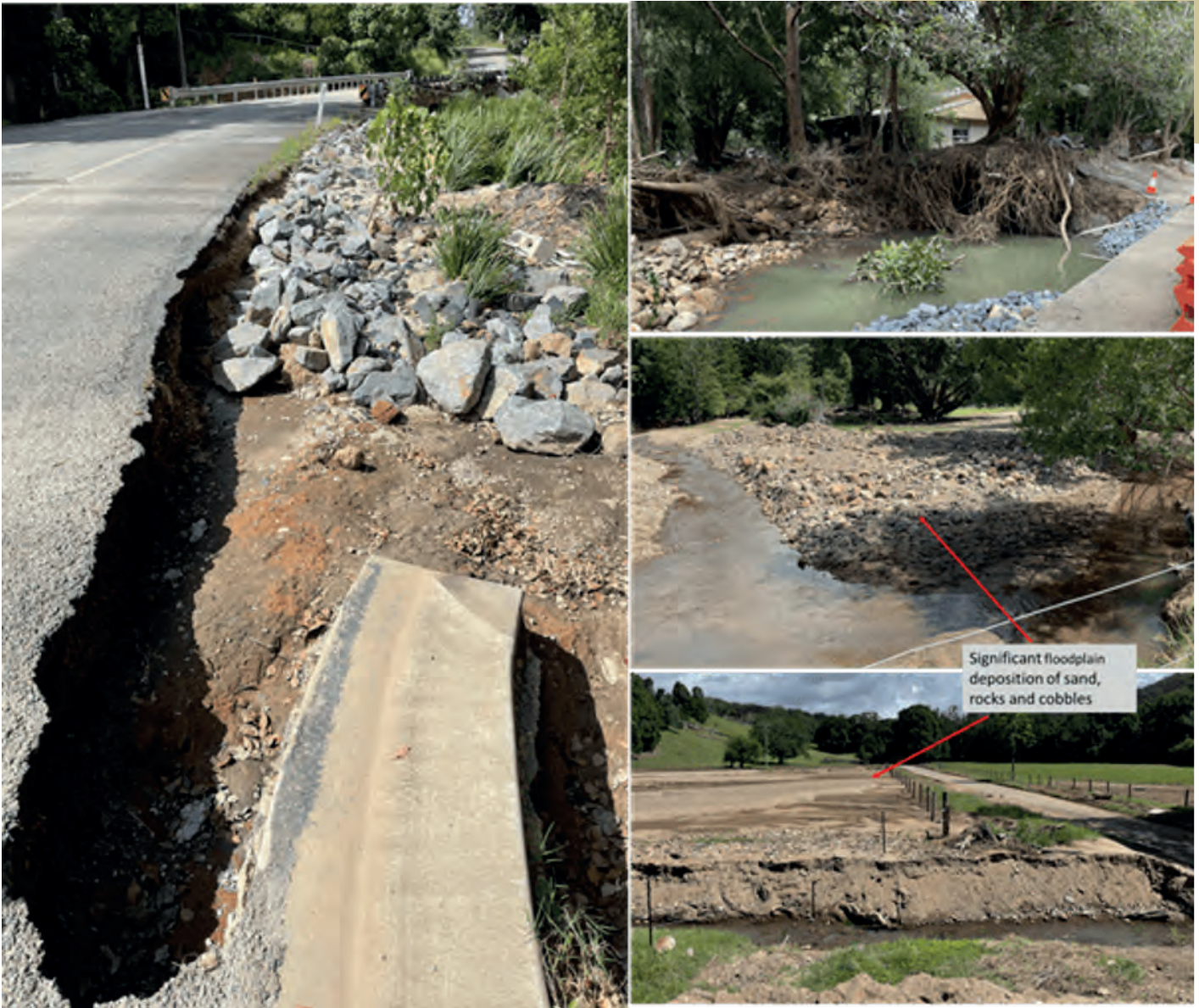
Figure 17: Road base and soil erosion from roadways and tree roots (left & top right) and evidence of fluvial geomorphic change with the deposition of sand, rocks and cobbles on floodplains (mid and bottom right) caused by deep and fast flowing flood waters in the confined Brunswick River catchment between Main Arm and Upper Main Arm. (Photo courtesy of Risk Frontiers 2022)
