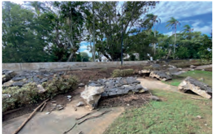
Figure 5: Examples of structural damage in the Lismore CBD. Clockwise from top left - stormwater drain and gutter, car park surface, a stone wall adjacent to the Richmond River and the rear bar of the Richmond Hotel. (Photo courtesy of Risk Frontiers 2022)
