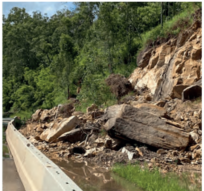
Figure 4: Washed out railway line (left) on Naughton Road between Casino and Lismore and a rockslide (right) closing one lane of Bentley's Road approximately 10km from South Lismore. (Photos courtesy of Risk Frontiers 2022)
