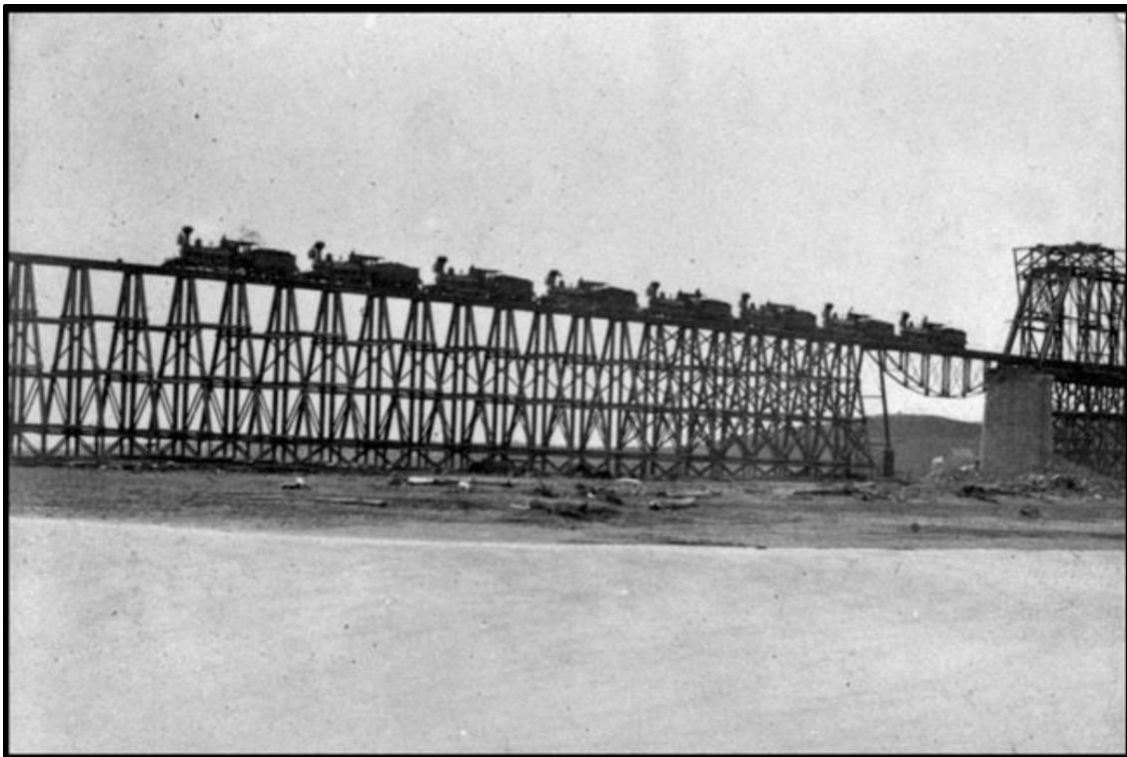
Figure 16: Photograph Taken during Weight Test of Historic Bridge on October 21, 1882, Showing Western Pier and Trestle Within the Ordinary High-Water Mark (Source Unknown).
