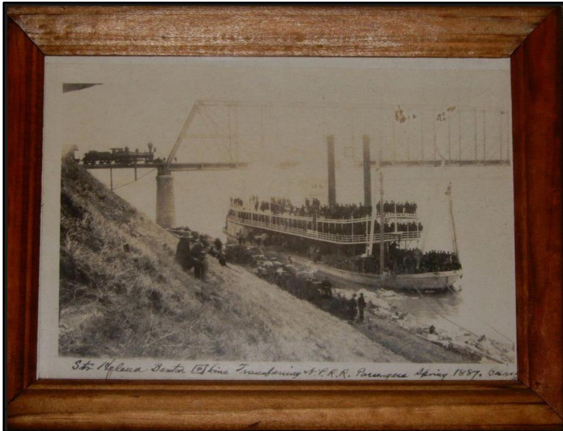
Figure 14: 1887 Photograph Showing Transfer of Goods from the Steamboat in Foreground to the Historic Bridge in Background with Pier 1 Within the Ordinary High-Water Mark (Copy of Photograph in Private Collection).
