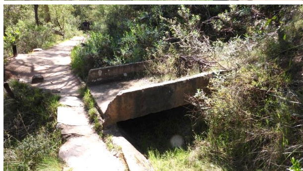
Gate (top) and silt-diverter over the water race (bottom) (Photos: Mark Watkins)
