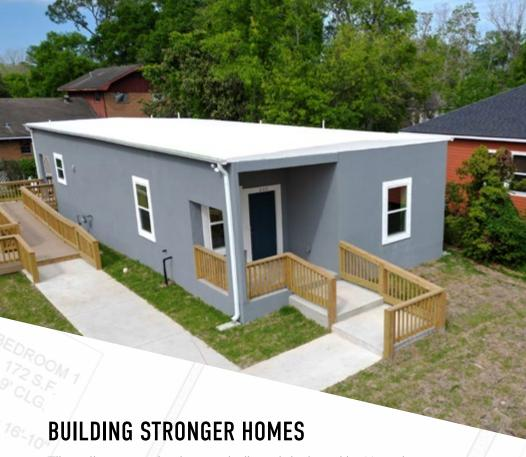
Tilt-wall construction homes, built and designed by Hercules Concrete Homes, use concrete for the slab, wall panels, and roof structure. This method is one of the fastest growing construction mediums available today. Tilt-wall construction offers homeowners a cost-effective, energy efficient, and durable residence with unlimited architectural versatility and appeal.
