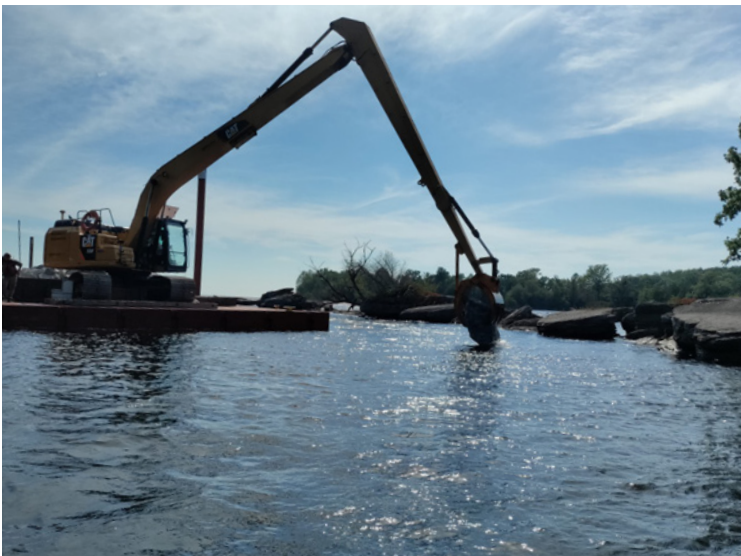
Construction crews work to create fish spawning beds in the Black River, a tributary to Lake Ontario, which will benefit walleye, a sportfish, and threatened lake sturgeon. Credit: U.S. Fish and Wildlife Service
