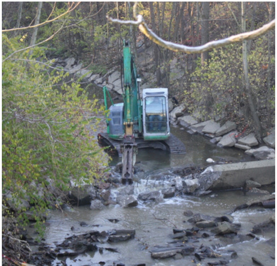
The removal of impediments to fish passage, such as dams, will allow for fish to more easily pass through Euclid Creek. This work has already happened in various parts of the Cuyahoga, including Baldwin Creek, pictured above. Credit: Soil and Water Conservation District
