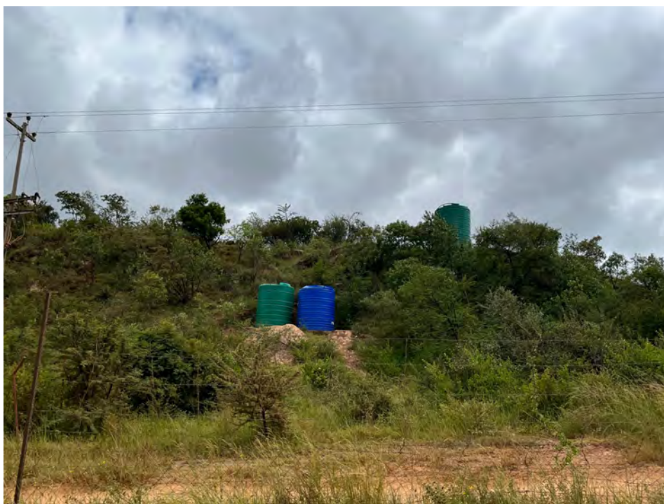
Photo 1: Water storage tanks and power supply on Happy Valley Claim
