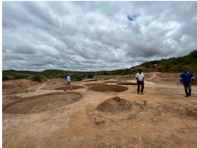
Photo 12 : Leach tanks on the tailings.
