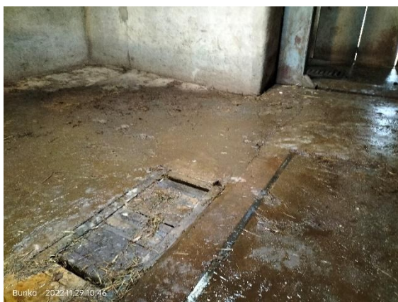
Fig. 26 – Gully cover and concrete floor
