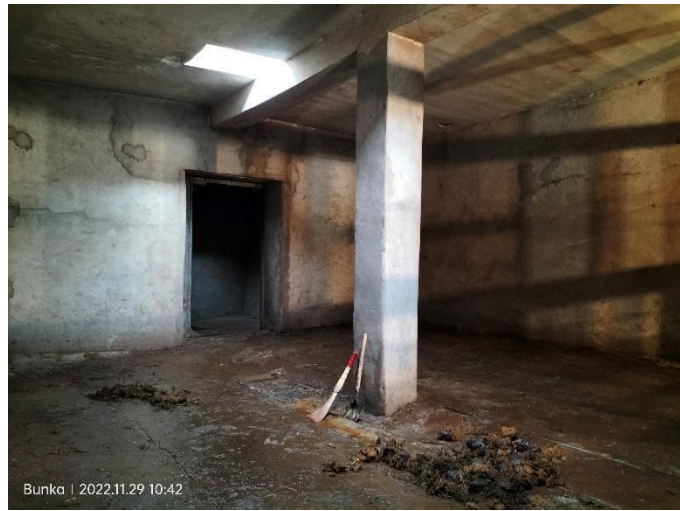
Fig. 21 – Skylight and construction type
