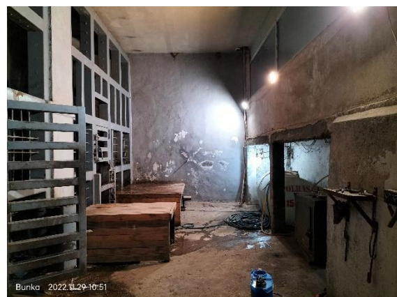
Fig. 17 – Staff corridor and flood lamps
