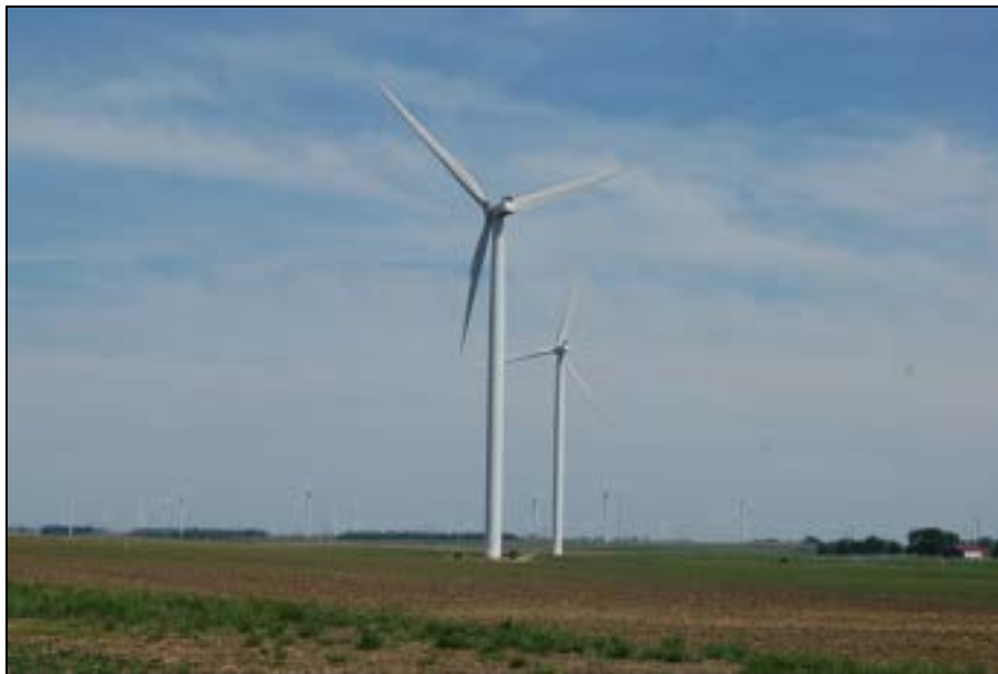
Figure 6: View of Wind Turbines located across N 2800 East Road looking southeasterly from the driveway.
