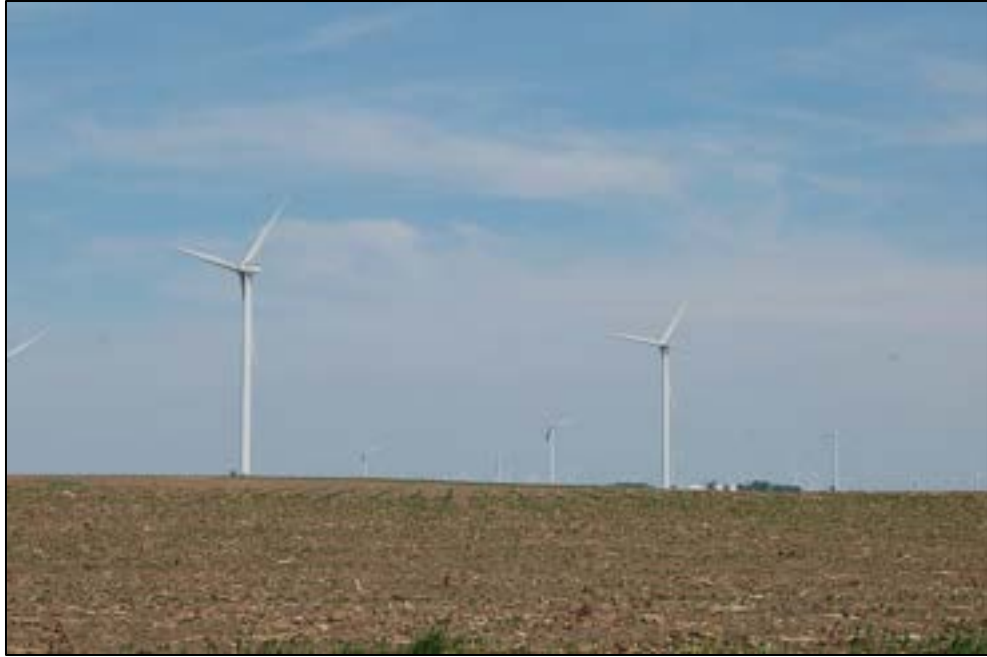
Figure 21: View of Wind Turbines across N 2900 East Road looking westerly from driveway entrance.
