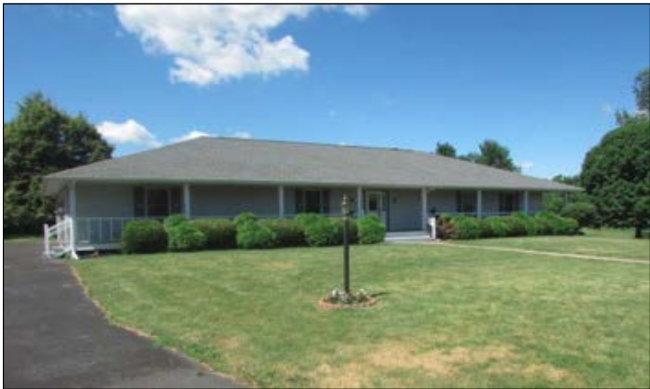
Figure 8: View of residence looking southwesterly from the edge of the driveway.
