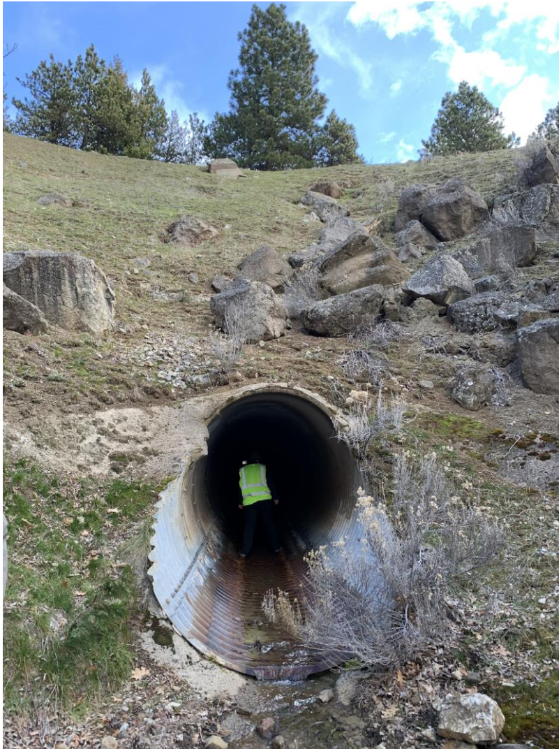
Figure 3-11. Bear Gulch culvert outlet with access road bench at top of the image. I-5 is not visible from the culvert outlet.
