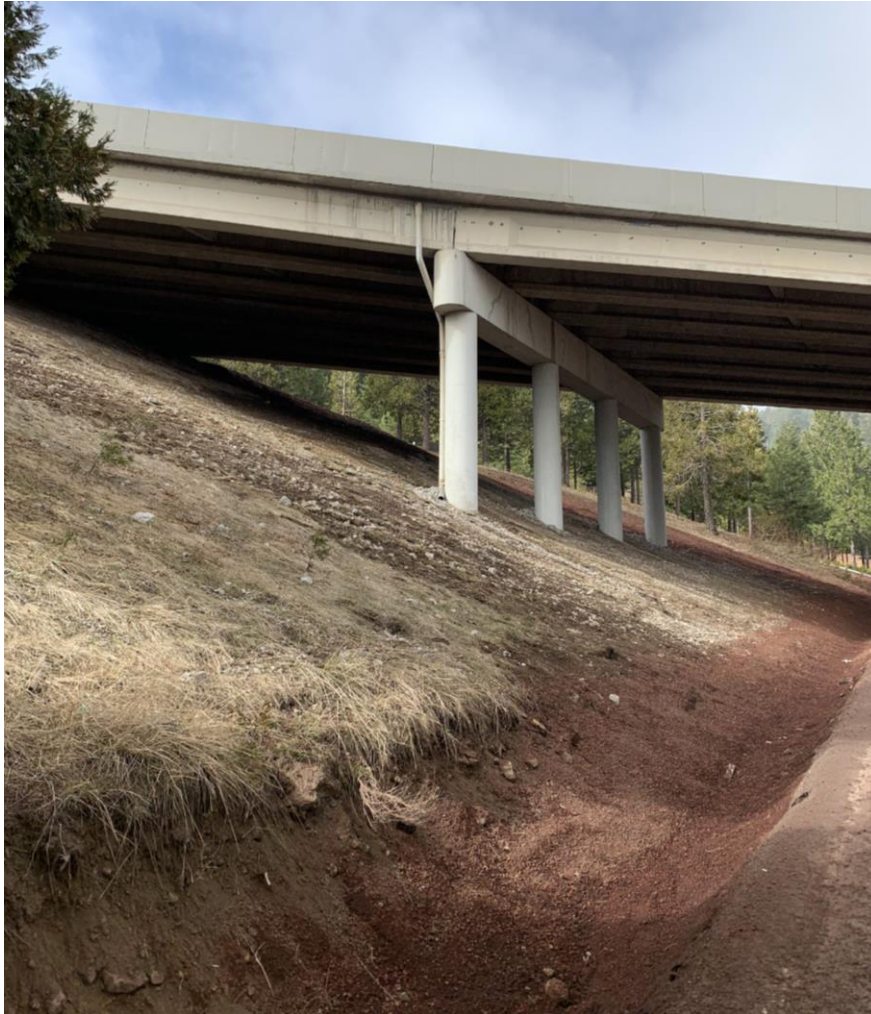
Figure 3-8. Mt. Ashland Exit bridge (southbound) (looking west).
