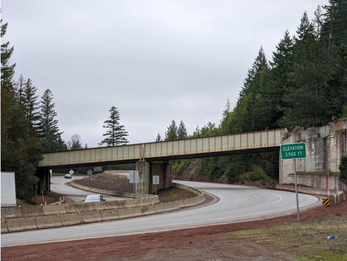
Figure 3-6. Wall Creek Railroad Bridge (looking south).
