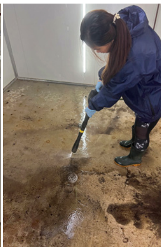
After the room is emptied, the next step is gross cleaning to remove soil and debris; start at the top and move down.
