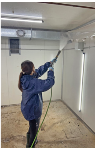
After the room is emptied, the next step is gross cleaning to remove soil and debris; start at the top and move down.
