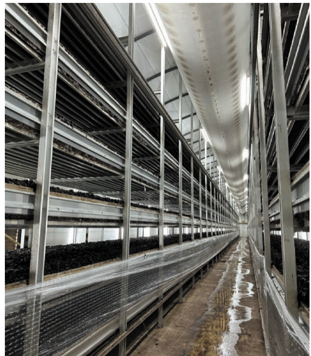
Rooms at Monaghan are a massive 60m long.
