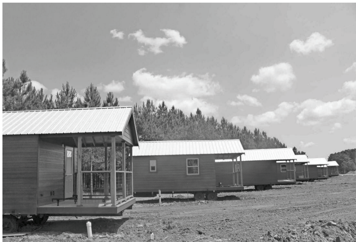
The cabins at In The Pines RV and Cabin Village, located near Winnabow, are in place and waiting to be tied down on May 11. RENEE SPENCER/STARNEWS
