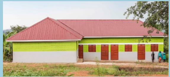
Staff Housing Reconstruction
