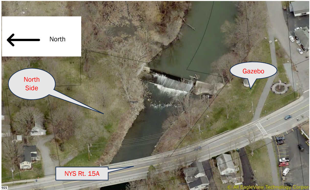
Figure 4. Veterans Memorial Park, Gazebo and dam (Aerial view toward the east)
