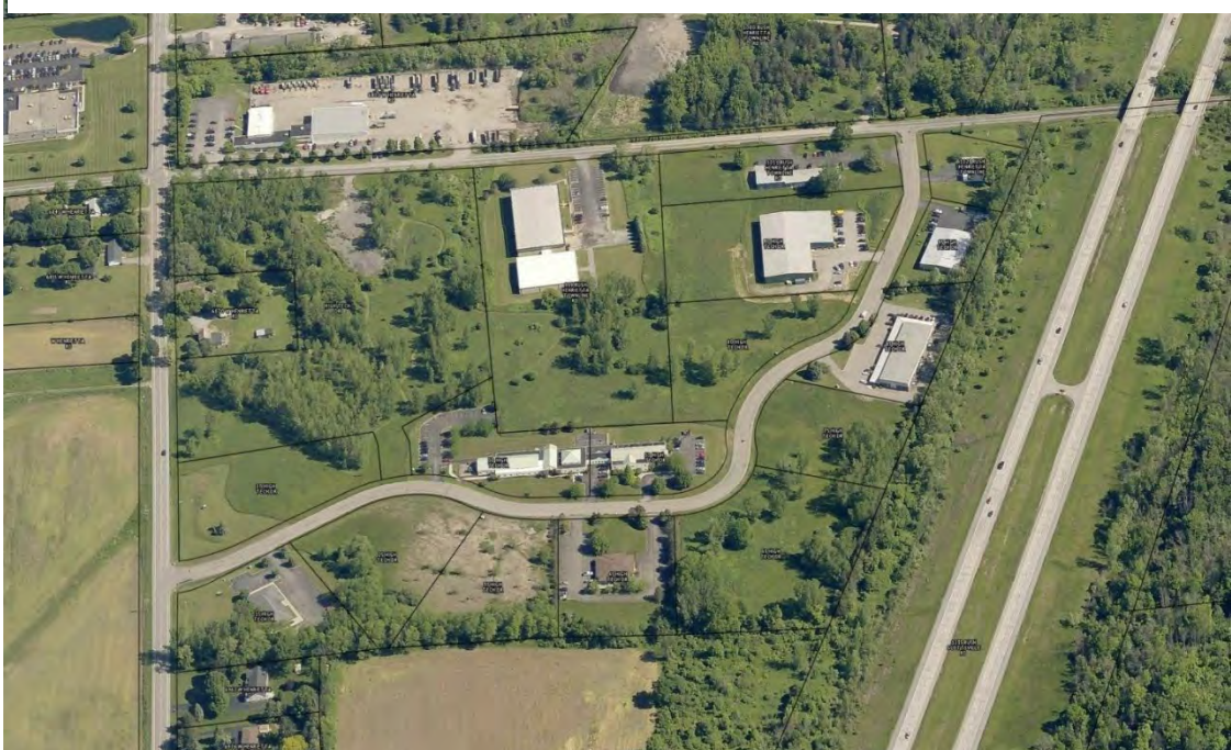
Figure 12: Business Park (High Tech Drive)
