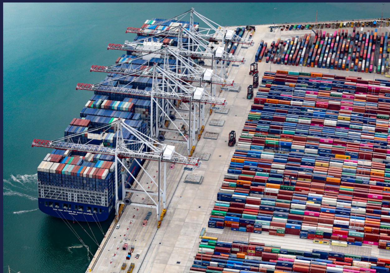
Aerial shot of cranes at DP World Southampton courtesy of DP World.
