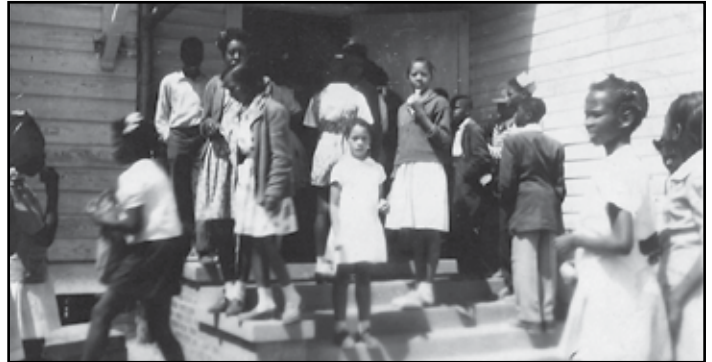
A typical two-room wooden school house like the one on Island Street.
