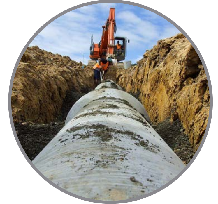
Pipe network upgrades
