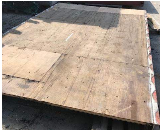
Figure 1: Image of the container floor.
