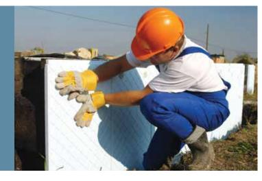
A test program conducted in August 2008 evaluated the field performance of expanded (EPS) and extruded (XPS) polystyrene foam insulation in a side-by-side, below grade application following a continuous 15-year installation period.
