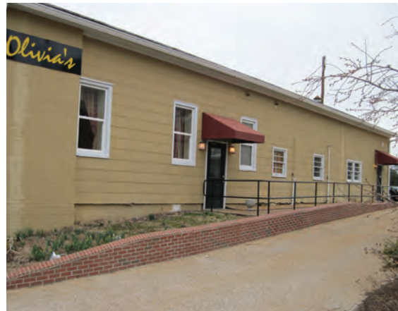
An accessible entrance through a well-marked side entrance, directly from a parking area, is a good solution for many buildings.
