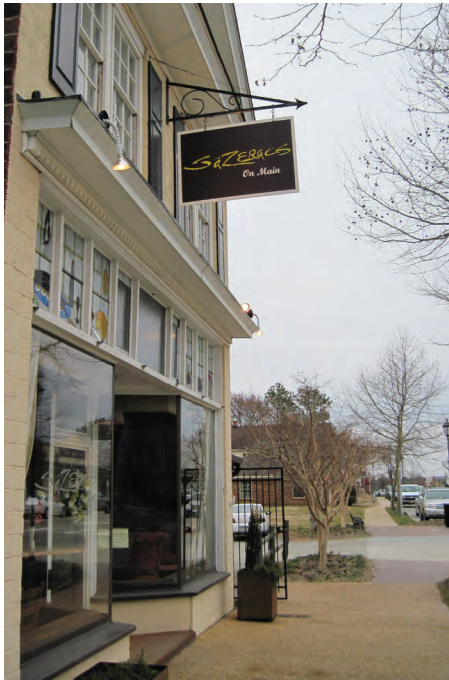
Many traditional mercantile buildings have no setback.
