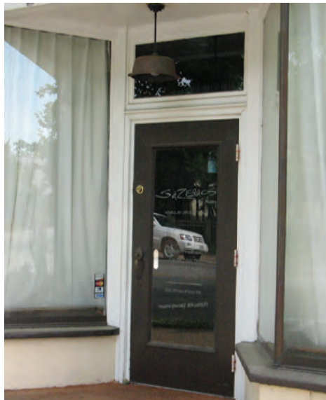
A recessed or hanging fixture at the ceiling of a recessed storefront is an appropriate way to light a storefront entry.
