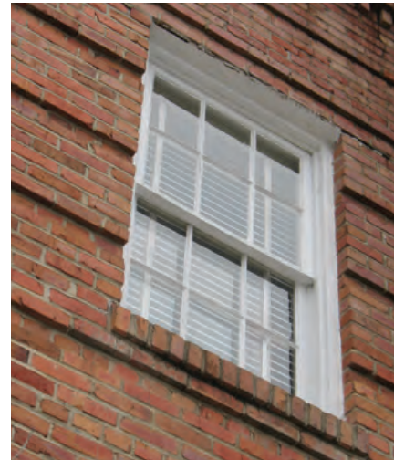
Wood double-hung windows, such as this example with a six-over-six divided light pattern, are common.
