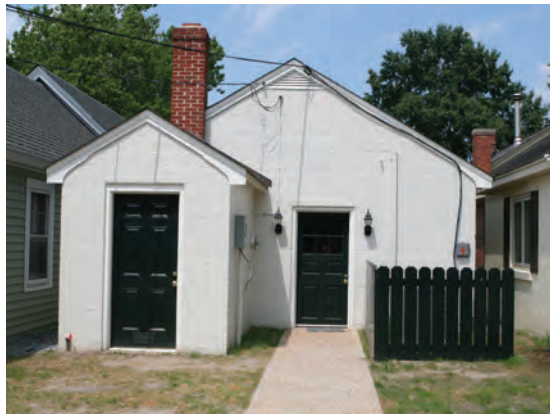
An existing business (top) planning to add mechanical equipment and using the rear entrance as access from parking can provide a painted wood and landscaped enclosure for utilities (above).
