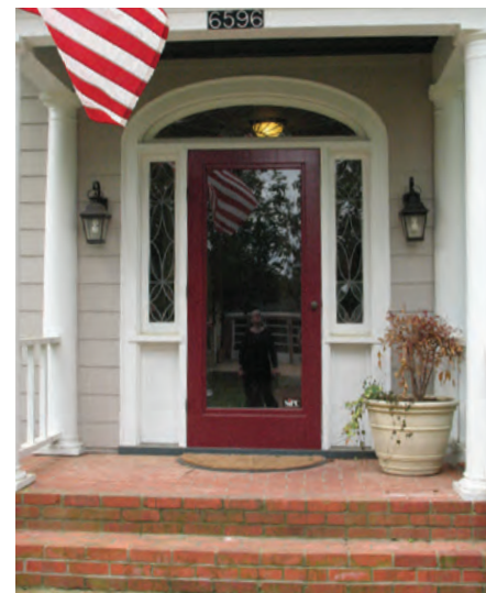
Decorative door trim, sidelights and transoms are character-defining features that should be retained.
