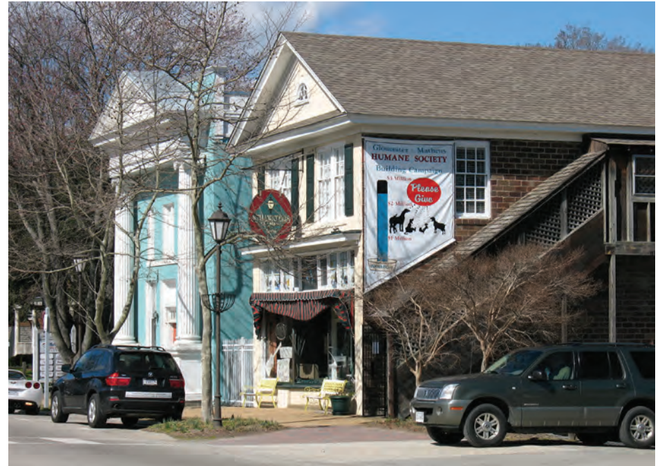
Early twentieth-century buildings on Main Street are a full two stories and are classically designed.
