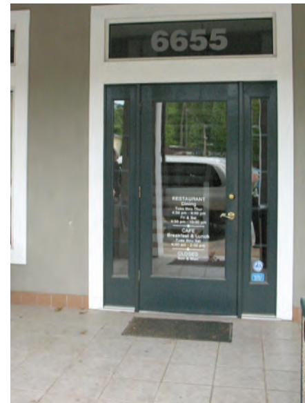
Full glass wood storefront doors are the most common and most appropriate doors in the Main Street area.
