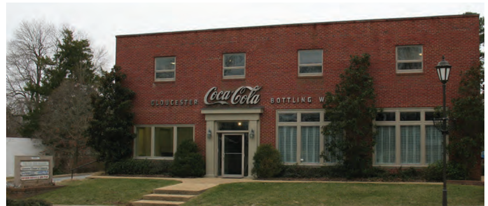
A wall-mounted sign of cut-out letters gives the historic name of the building. Tenant signage is posted on a freestanding monument sign.
