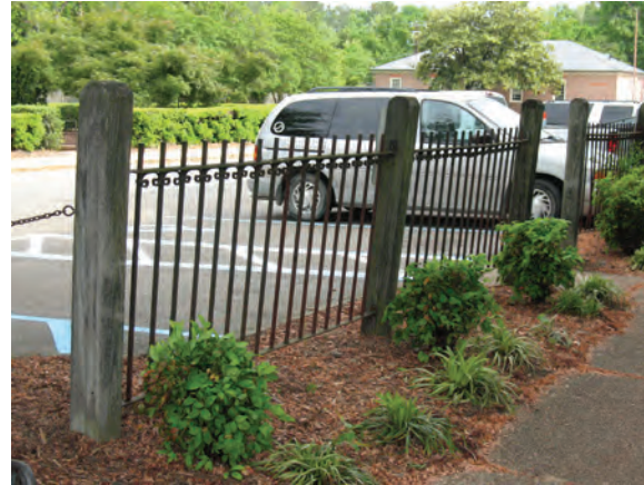
Wood posts support an iron decorative fence to provide an edge to a parking area.
