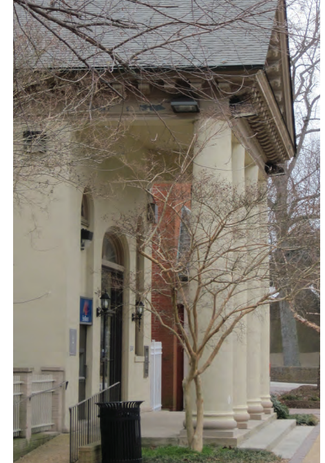
Traditional non-mercantile buildings in the district often have classical porticos, which function in a similar way to an awning or a canopy, protecting customers from the weather and creating an outdoor gathering space.
