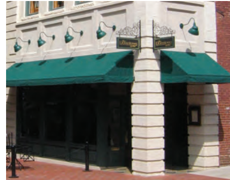
Gooseneck fixtures highlight this building's awnings.
