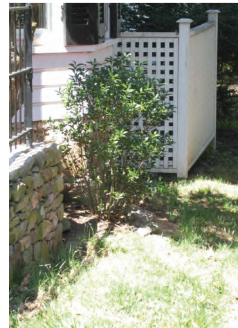
A lattice fence provides a screen for mechanical units.
