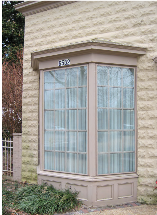
A common feature on many Gloucester Main Street buildings is the bay window, which extends into the front setback zone and provides a display area.
