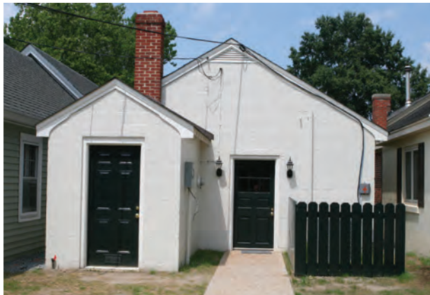
A photo of the completed project shows how an accessible entrance from the rear parking area has been made more inviting with restored doors, an enclosure for utilities, paint, and lighting.
