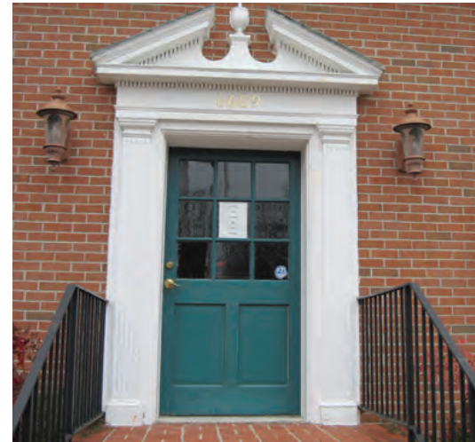
Wall-mounted lights beside a building entrance are common throughout the village.
