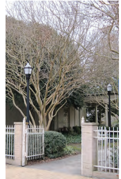
Traditional acorn style fixtures are used here to light a path through a courtyard space.
