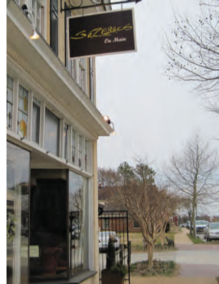
This traditional storefront has a recessed entry, decorative transom windows, and a storefront cornice.
