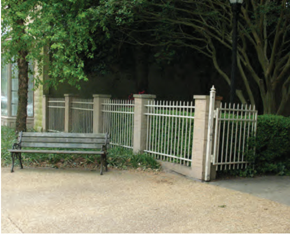
Brick piers combined with metal fencing enclose a courtyard space.
