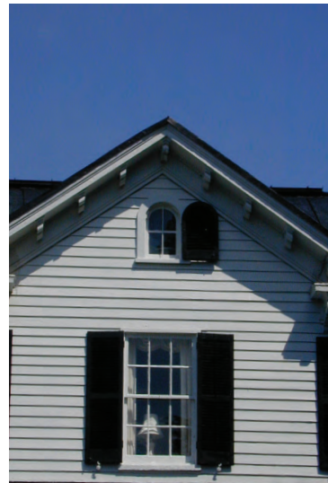
Shutters should be the same shape and size as the opening they are intended to cover.
