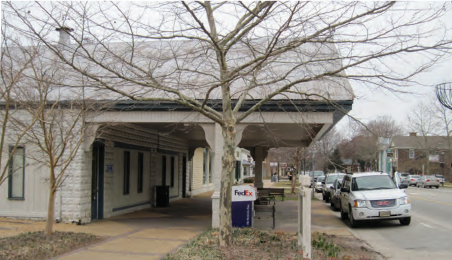
A deep canopy that is actually an extension of the gable roof provides a covered place for street furniture.
