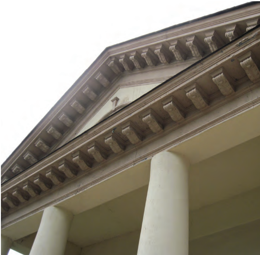
Metal is commonly used on decorative elements on historic buildings, such as this cornice and pediment.
