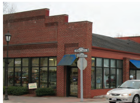
Parapet walls on mercantile form buildings can range from very simple (above left) to more decorative, such as the stepped, corbelled brick example at left.
