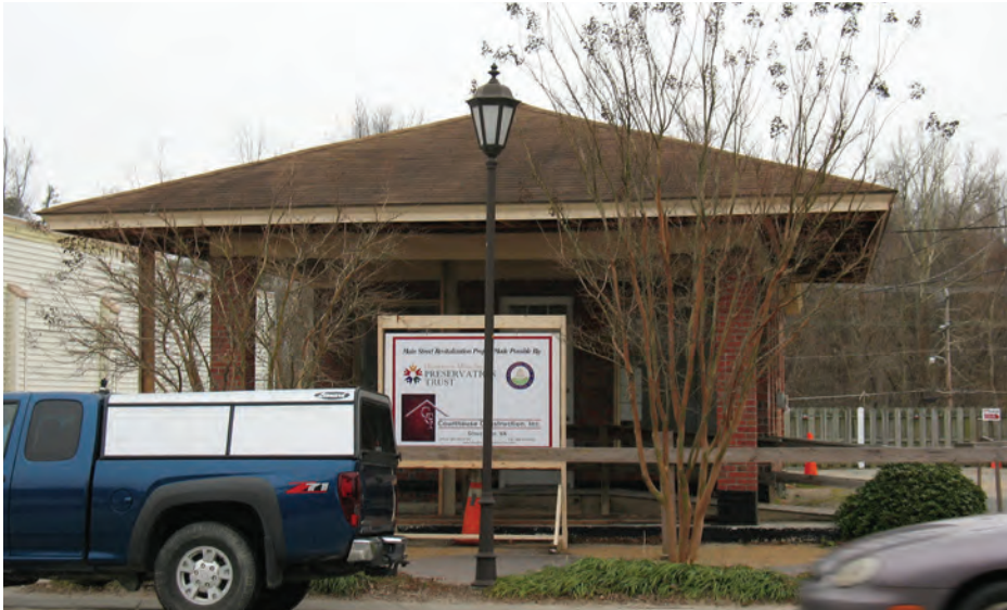
Auto-oriented building forms are more common towards the east end of the Main Street area and sometimes include a porte cochere.
