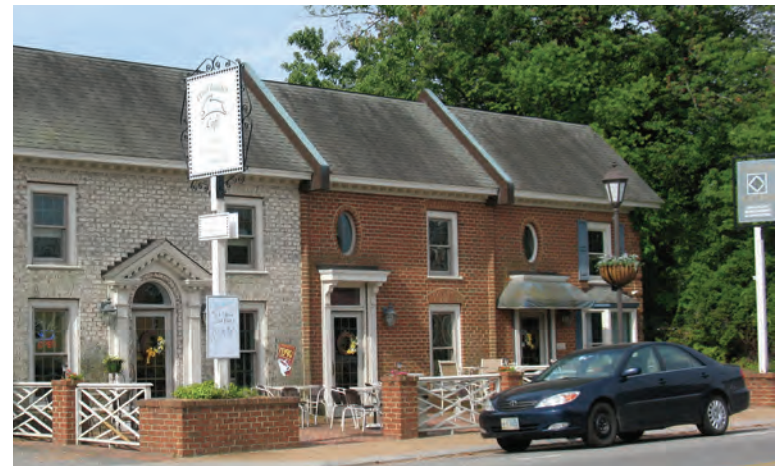
Roof forms and materials in the Main Street area vary greatly, creating a variety and texture that is unique to the village. In the top view above, many different forms can be seen; in contrast with the view below, a row of buildings with the same roof form creates continuity.
