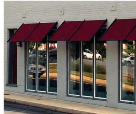
A modern awning shape on this building is finished in a color to match the doors.
