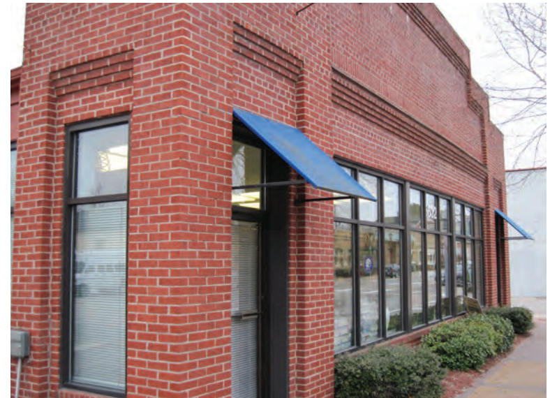
A more contemporary storefront is decorated with corbelled brick accents.
