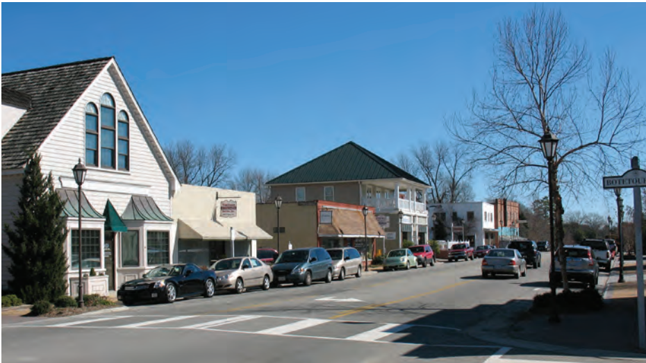
The variation of building size, setback, and style creates the unique village character that defines Gloucester’s Main Street.
