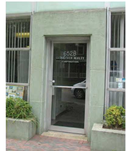
Aluminum storefront doors may be appropriate for modern buildings. Placement of wood doors with aluminum is not appropriate.
