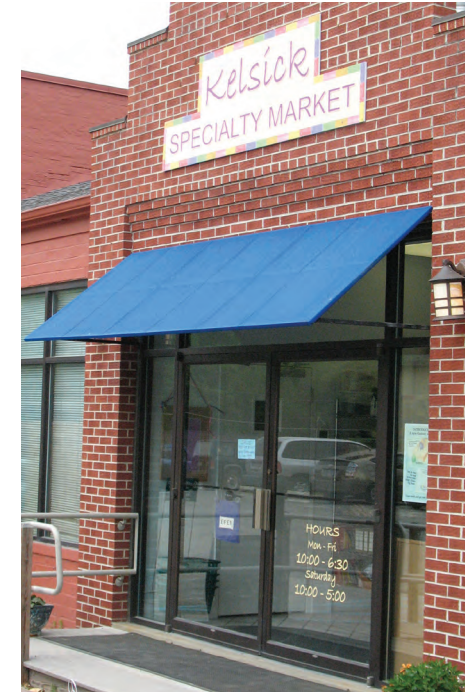
A more modern sloped fabric awning with open sides is appropriate for this facade.
