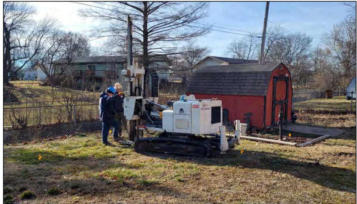
Use of small drilling rig to minimize damage to yards
