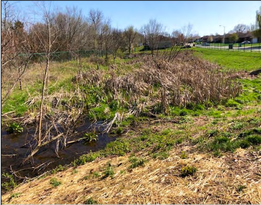
Existing stormwater basin conditions (April 2018)
