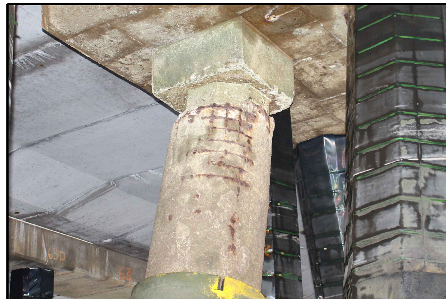
PHOTO 9, TYPICAL PILE TYPE C
