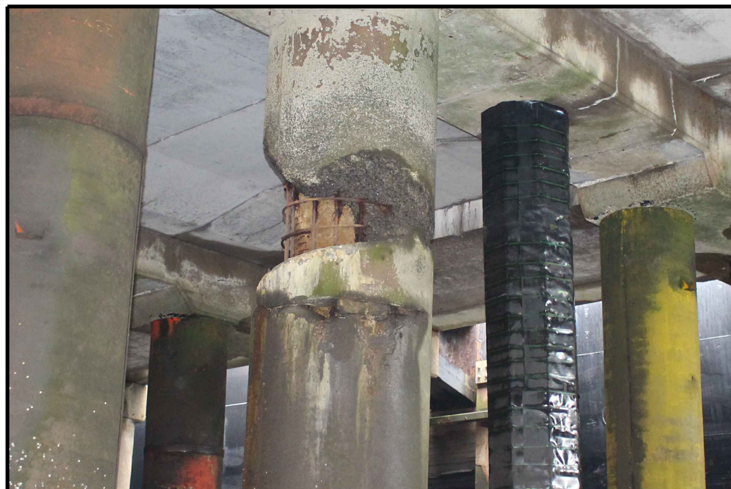
PHOTO 8, TYPICAL PILE TYPE B
