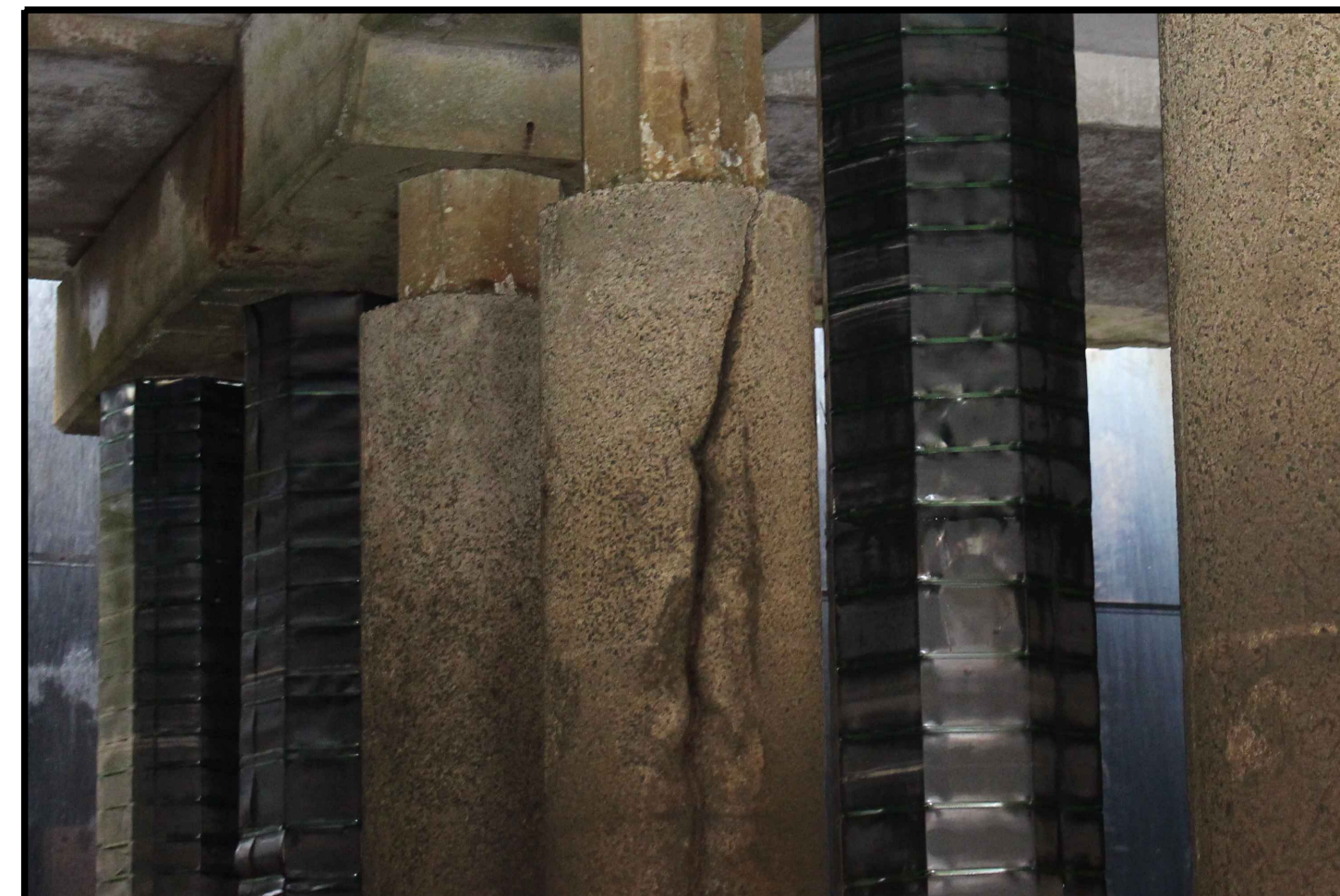
PHOTO 7, TYPICAL PILE TYPE A
