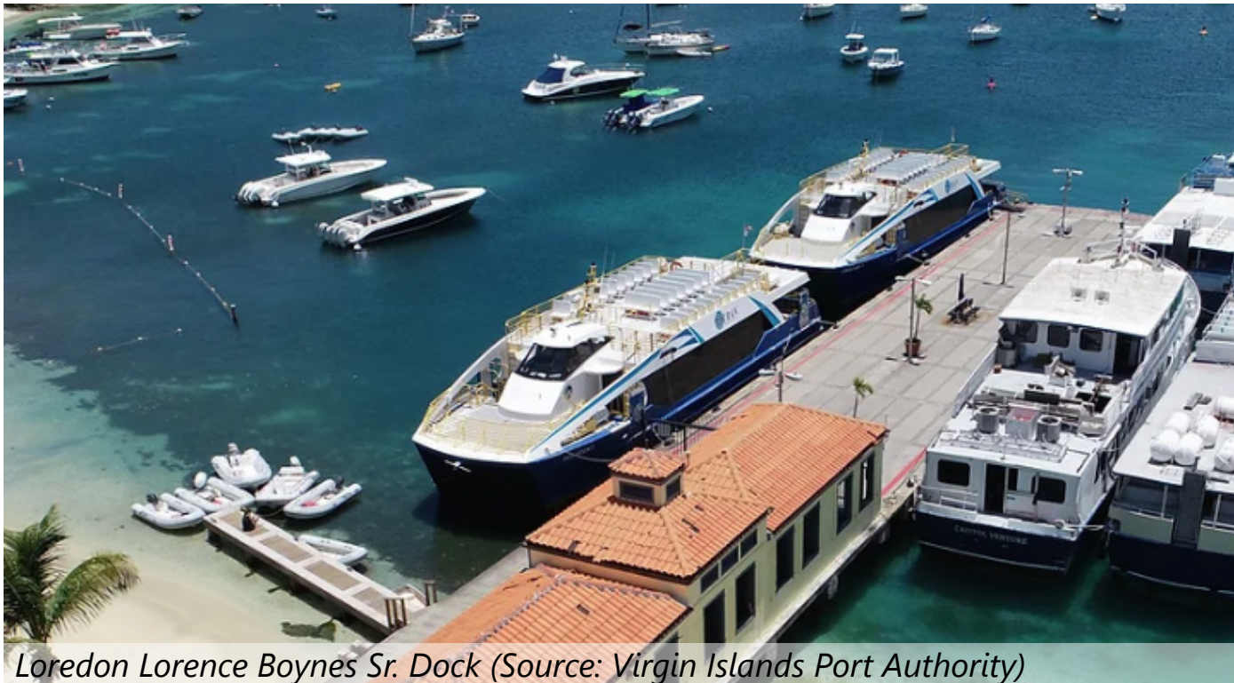
Laredon Lorence Boynes Sr. Dock (Source: Virgin Islands Port Authority)
