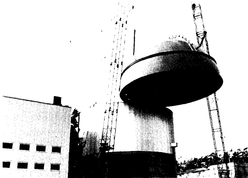
The dome of the KNK containment is swung into place (1967).
