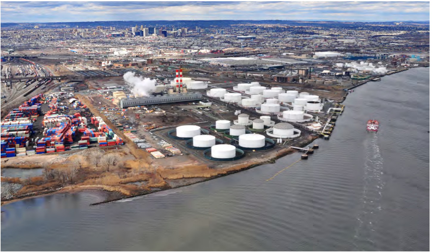
An aerial view of a biodiesel refinery and shipping facilities on the Passaic River waterfront with Newark, New Jersey, in the background.
