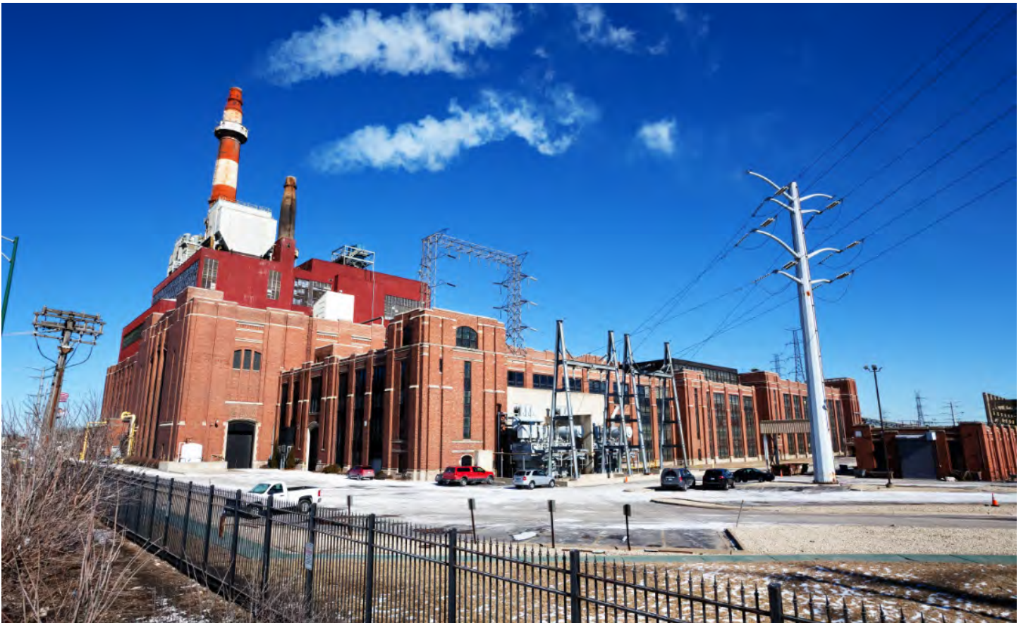
The coal-fired Crawford Generating Station in South Lawndale, Chicago. Demolition of the plant began in 2019. On April 11, 2020, the concrete smokestack was imploded, blanketing the nearby Little Village neighborhood with toxic dust.
