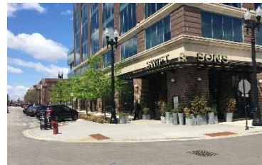
Curb Extensions / ADA Upgrades
