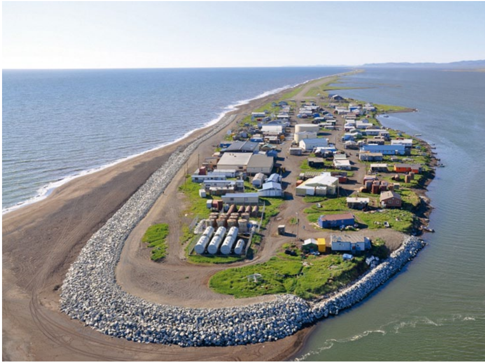
Photo 17.1: Shoreline erosion in Kivalina, Alaska.
