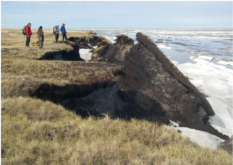
Photo 17.3: Permafrost thaw and shoreline erosion in the Bering Strait region.
