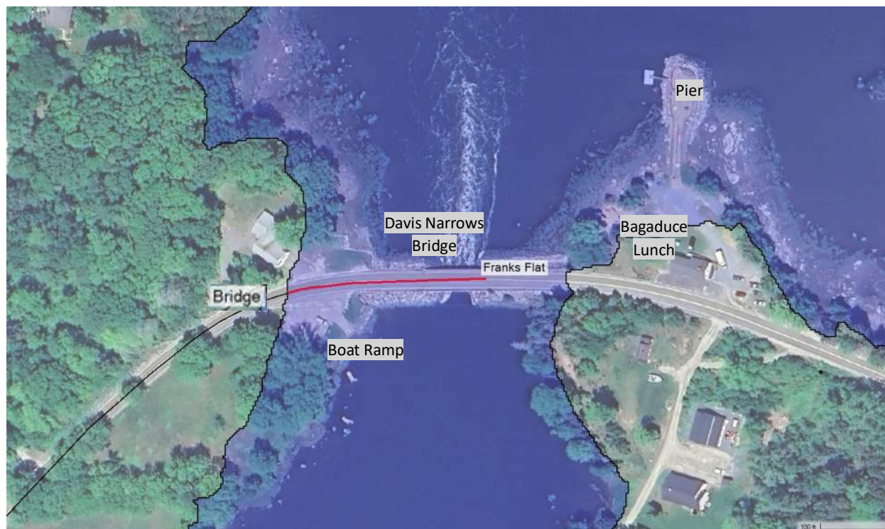
Figure 4-7. Bridge Road and Davis Narrows Bridge Inundation
