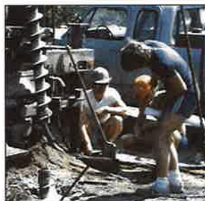
Installing a monitoring well, Washington County, Maine.
