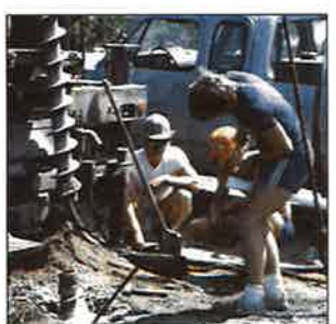
Installing a monitoring well, Washington County, Maine.
