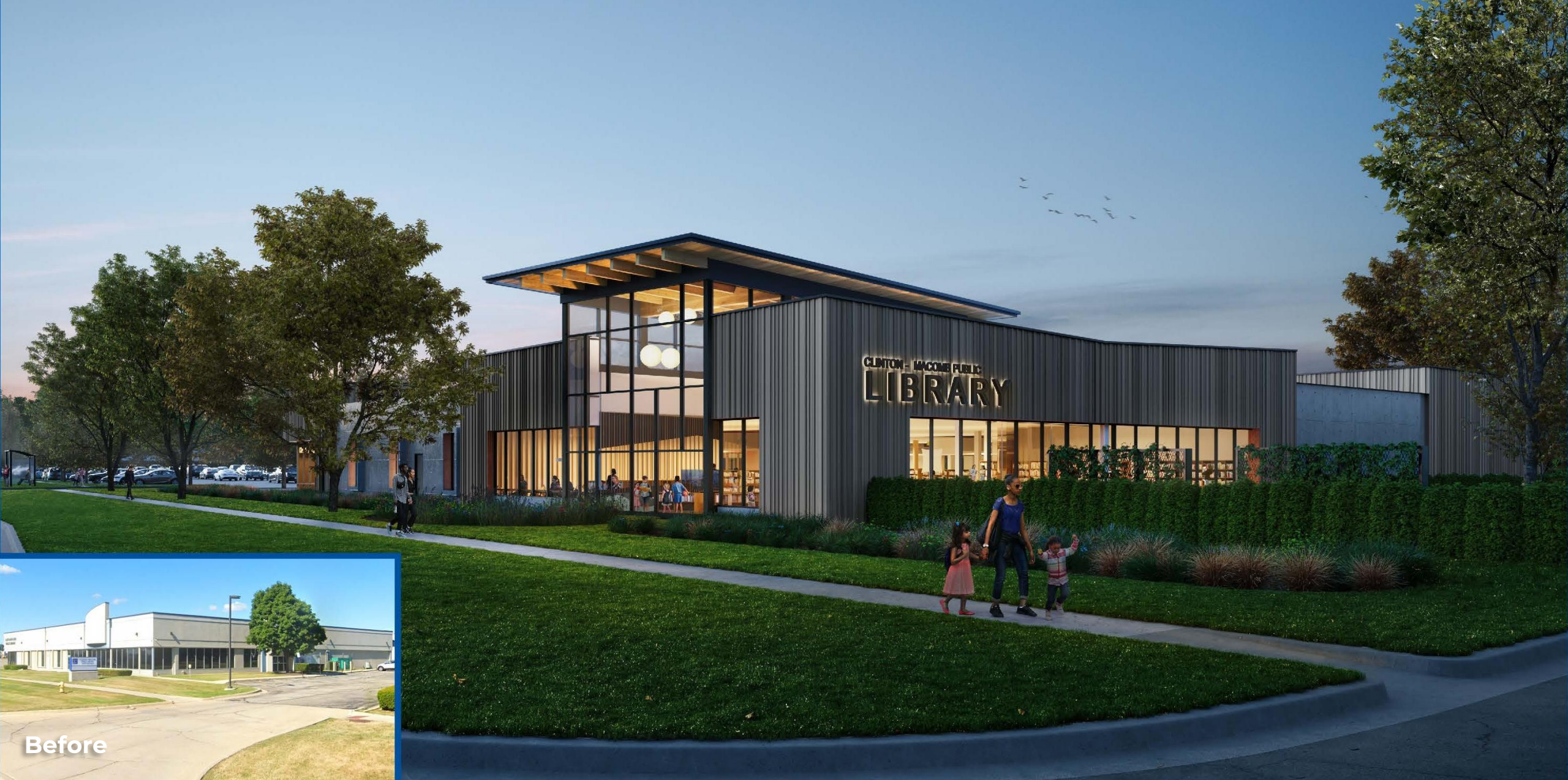
South Branch, Clinton-Macomb Public Library Macomb County, Michigan
