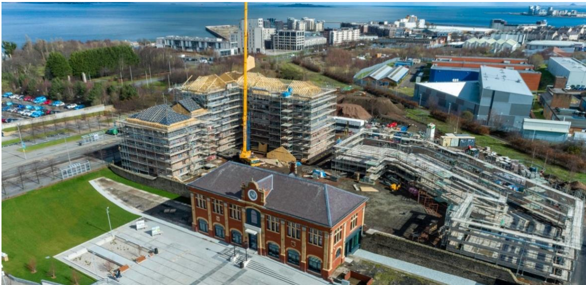
Figure 7: Pilot 1 Granton Site D1 On Site
