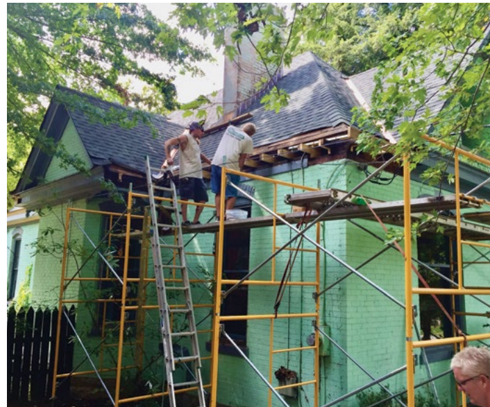
Replacing the roof and repairing the box gutters were priorities for Nathan Rouse's first round of Kentucky Historic Tax Credits.
