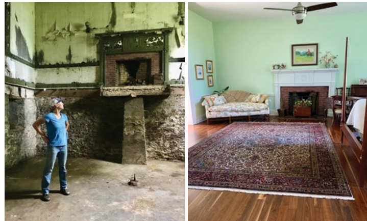
Here Anna-Coleman is standing in the basement below the master bedroom-to-be. The flooring as well as the floor joists were so damaged they had to be removed. The master bedroom today has walnut flooring which was installed throughout the first floor. The wood came from Anna-Coleman’s parents’ farm in Woodford County.
