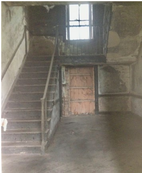
The entrance hallway after the initial restoration work and trash removal had begun and the same view after renovation. Anna-Coleman scraped and sanded the ash stair steps, which are original.
