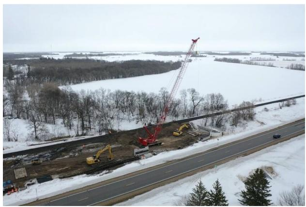
A construction crew works on a project to replace a series of culverts on a railroad crossing over the Middle River with a bridge near Newfolden, Minnesota, in the winter of 2023. The work marks the first component of a flood control project to remove part of the city of Newfolden from the 100-year floodplain. The second component of the project requires funding from the Minnesota Legislature before work can begin. Contributed/Morteza Maher
