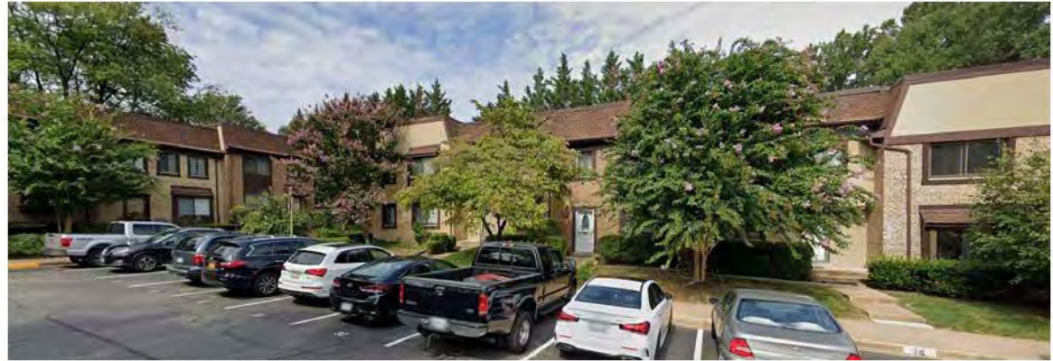
JERMANTOWN ROAD (ON MOTOR COURT)
