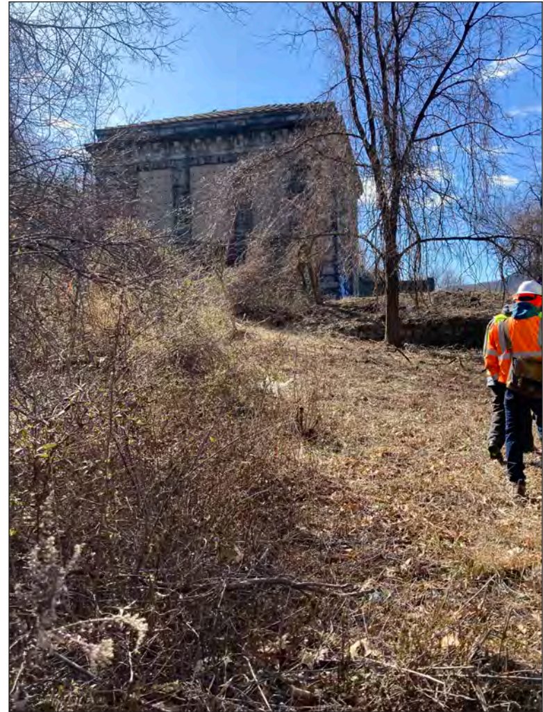
Bridge landing area on DEP site facing south 13
