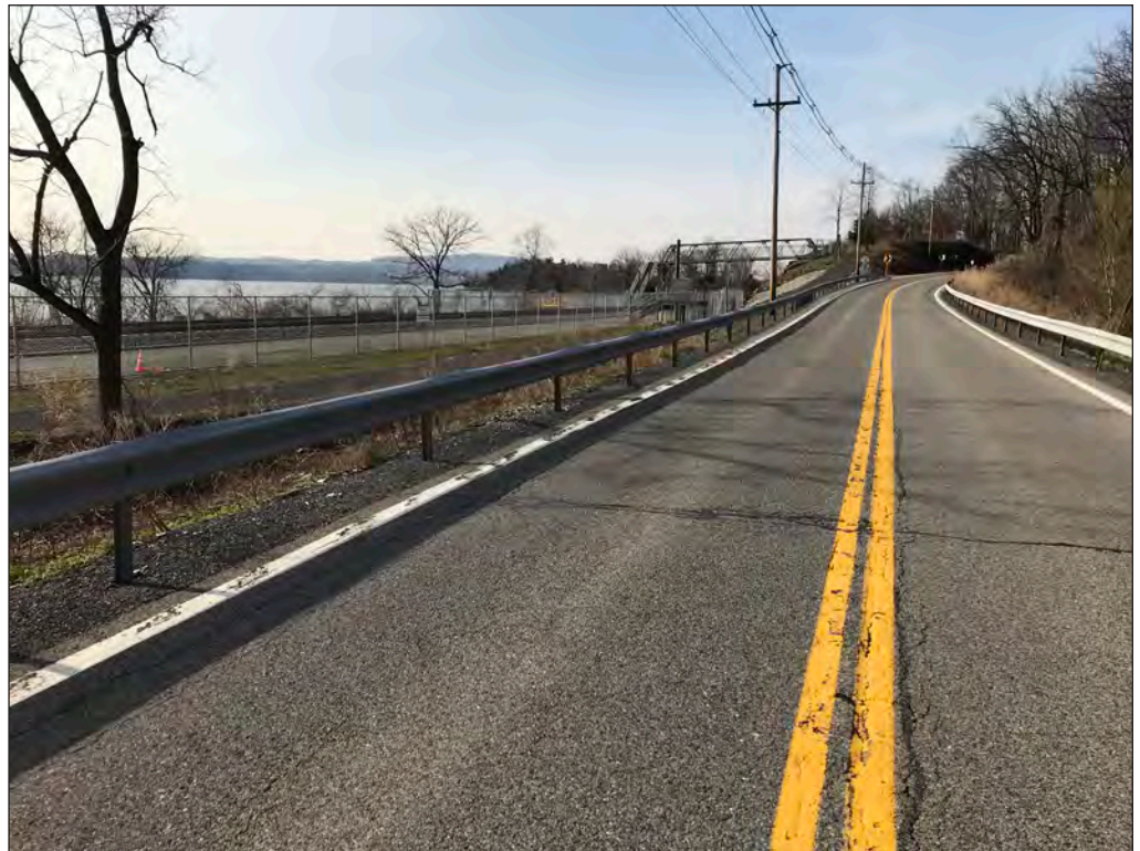
View from north end facing north 3
