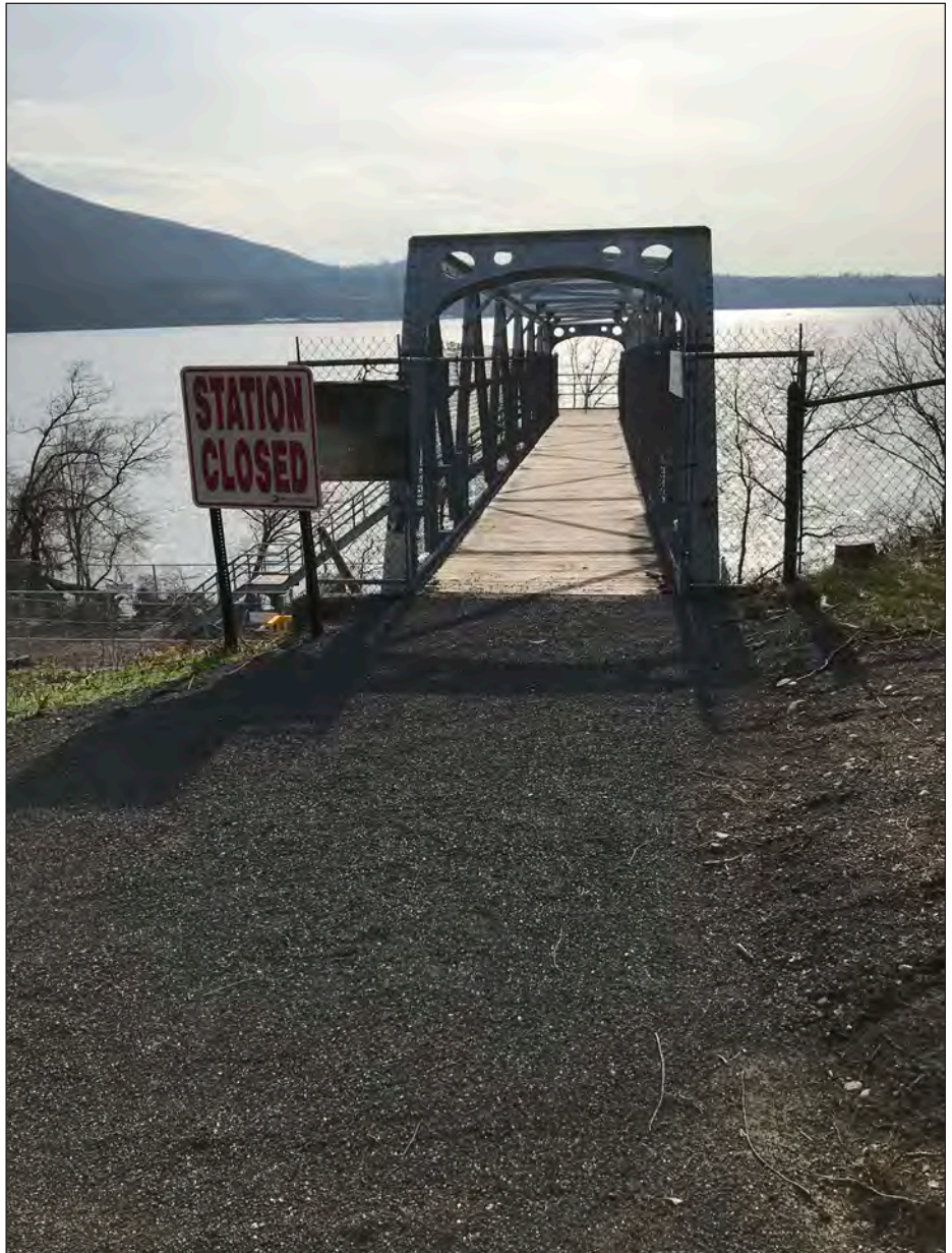
View from footbridge to train station facing west 1
