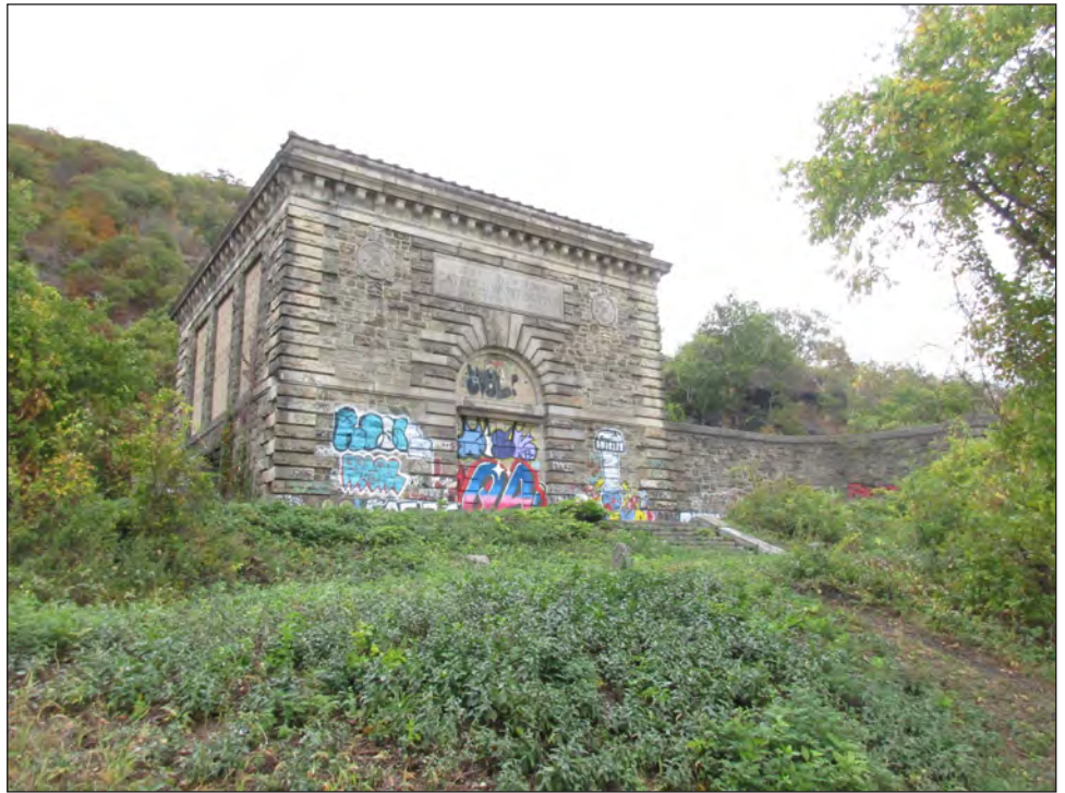
DEP building and trail location facing southeast 14
