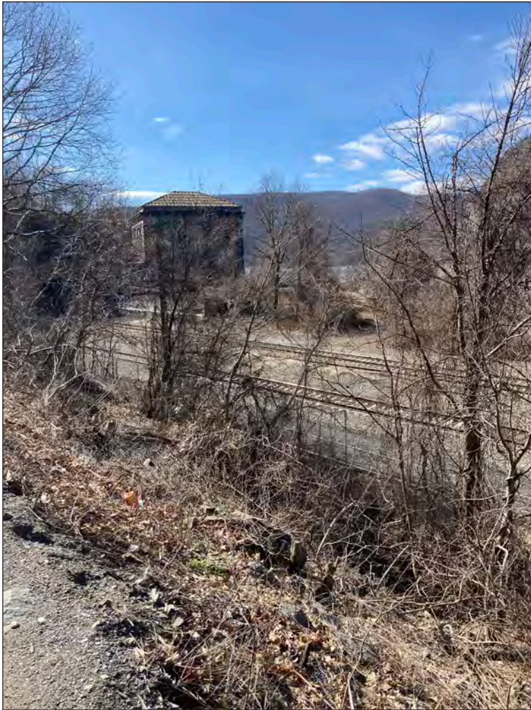
Approximate location of bridge east end facing southwest 12
