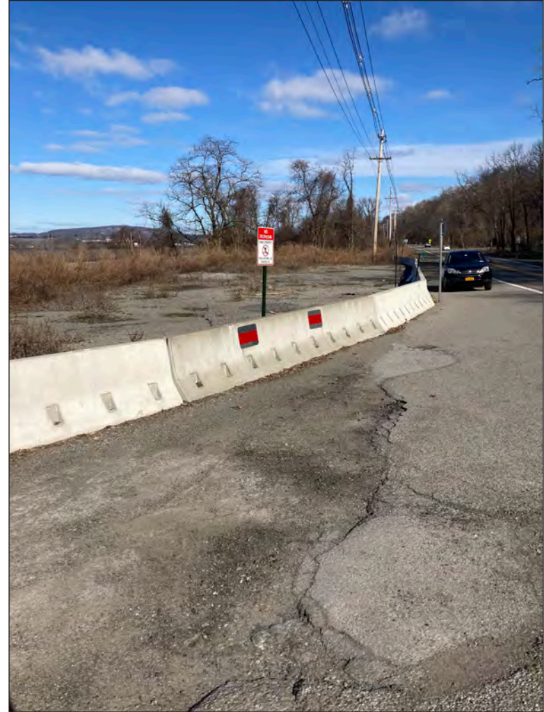
Closed off MNR parking lot facing north 11
