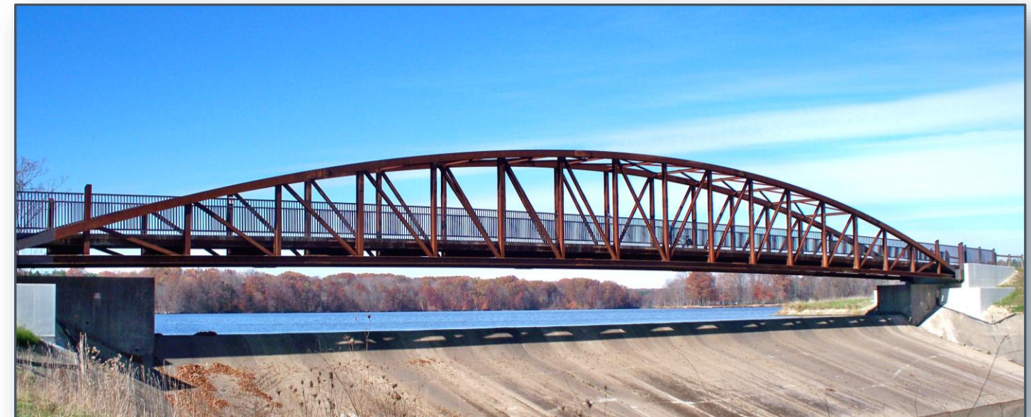
U.S. Bridge Seneca Bow-String Truss
