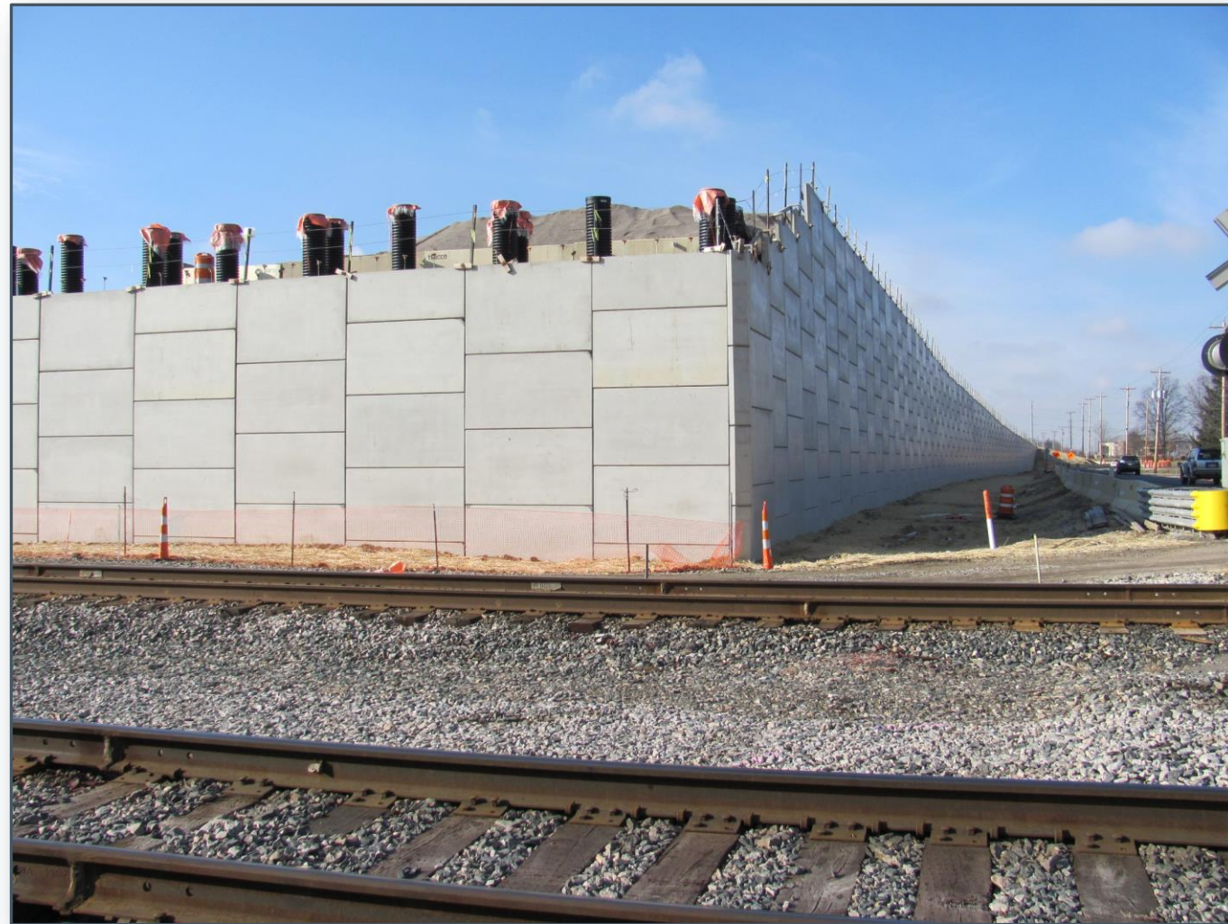
Tensar ARES® MSE Retaining Wall System
