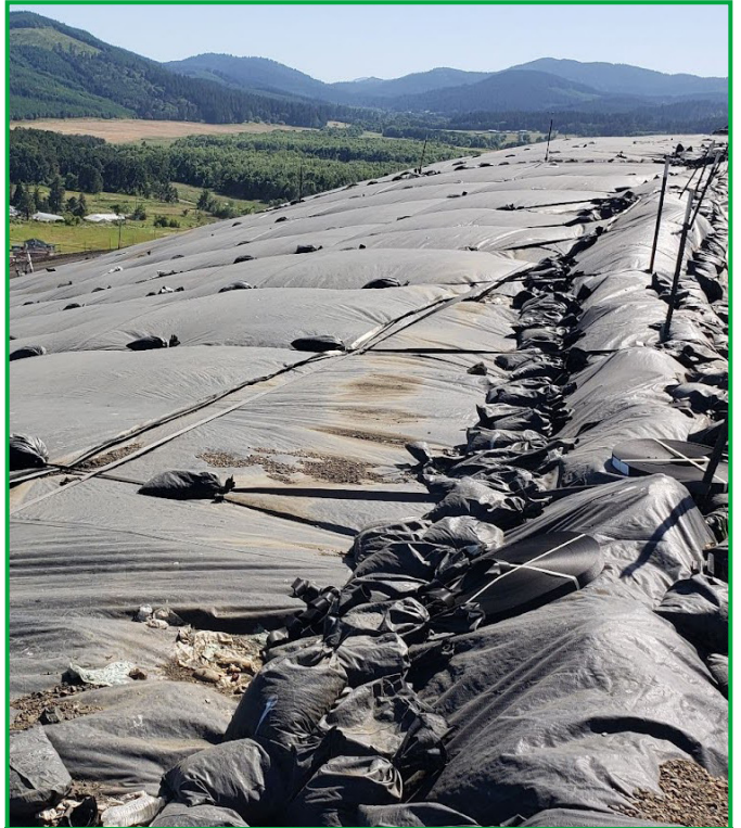
Photo of gas buildup on tarp, Coffin Butte Landfill, Corvallis, Oregon Image credit: EPA Inspection Report
