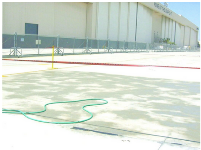
LEFT: Surtreat treated surface acquires a slightly darker, shiny appearance.
