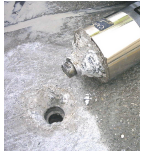
ABOVE: After application plug doesn't crumble, showing improvement.
