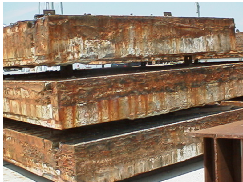
BELOW: An example of the corrosion that appears on metal elements at the launch pad.
