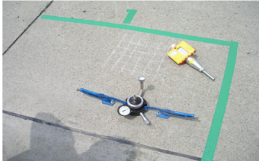
Permeability and Rebound pre-testing Area 1
