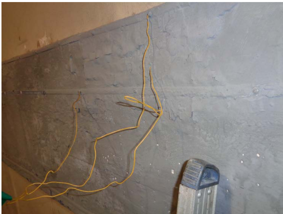
Figure 10 - Section 2 of the ring girder at Building 306 in the Naha Military Port, 2016
