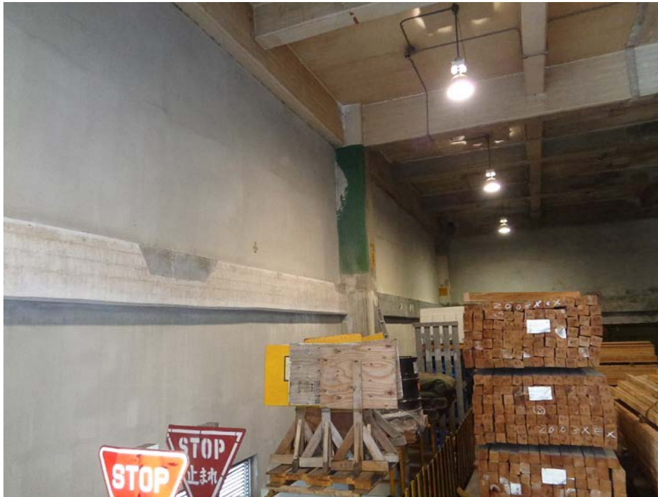
Figure 9 - Section 1 of the ring girder at Building 306 in the Naha Military Port, 2016
