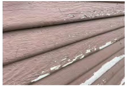
(Above) Typical “teardrop” profile clapboards on cottages observed during the field survey.
