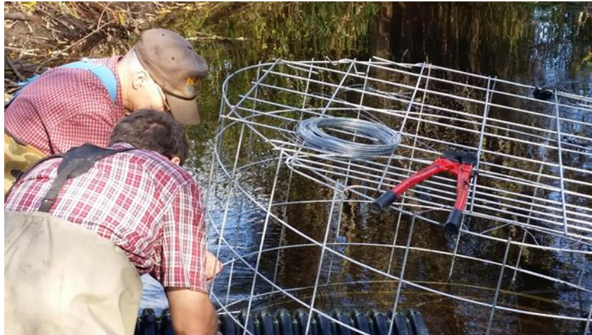
Photo 2. Installation of a fence and flow device along Chimacum Creek.
