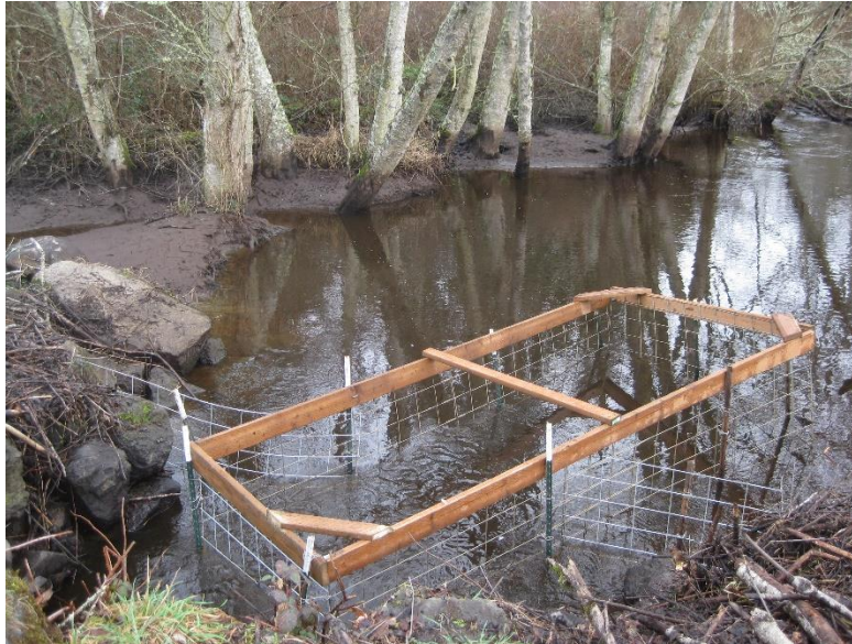
Photo 1. Beaver deceiver installed to protect culvert along Chimacum Creek.
