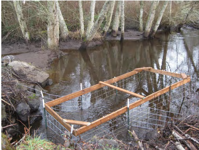
Figure 11. Beaver deceiver installed to protect culvert along Chimacum Creek.
