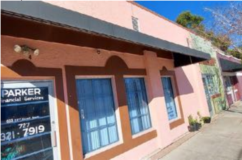
The former Twenty-Second Street Package Store. Photo courtesy of Ennis Davis, AICP.
