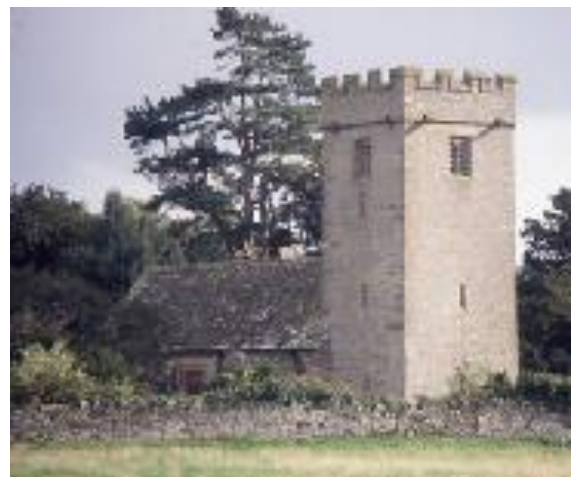
The 'forlorn window' is only slightly below the belfry window and clearly belongs to an earlier phase of construction.
