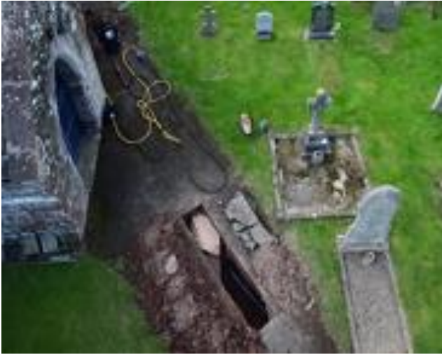
The foundations of the demolished wall of the north aisle, seen in the 2019 pipe trench
