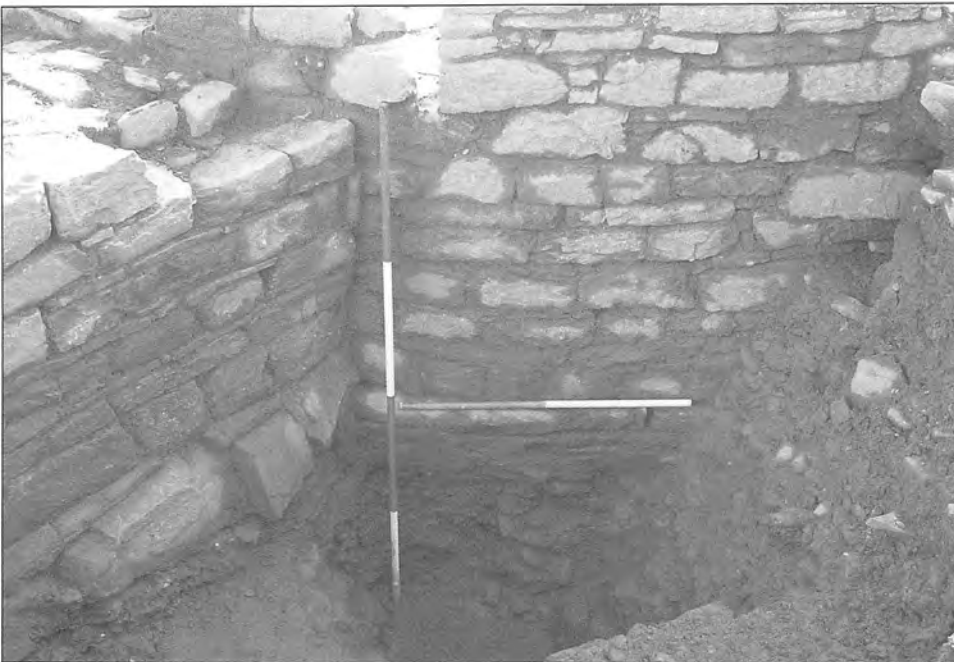
Plate 4 View looking S.E. showing foundations of semicircular tower (501).
